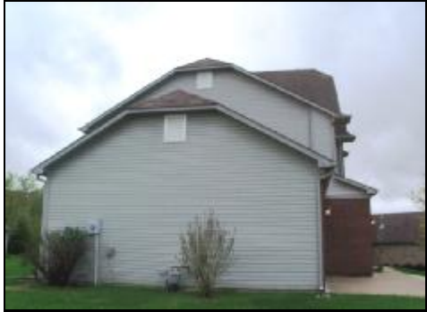
North side of home
