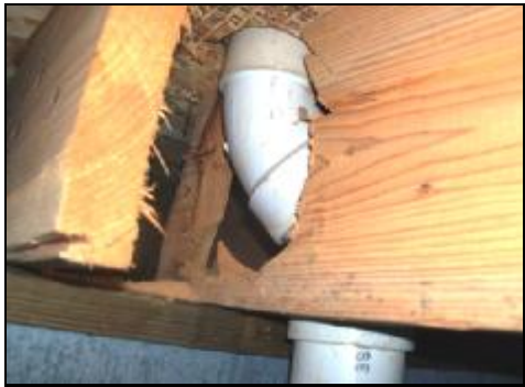
Cut out floor joist (under 1/2 bathroom)
