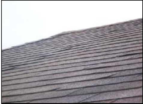
Roof II (shingle lifts)
