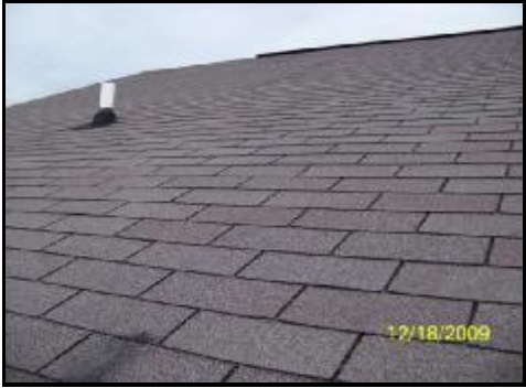
Roof III (rear)
