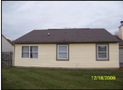
West side of home
