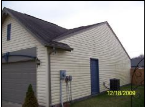
North side of home
