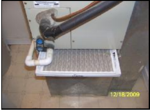
Furnace filter location
