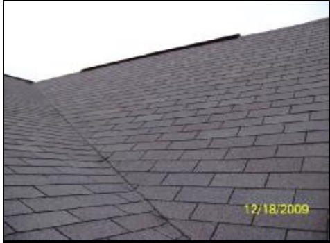
Roof I (front valley)
