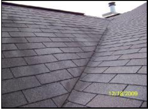
Roof II (front valley south side)
